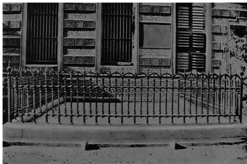
BLACK HOLE, CALCUTTA. ADJOINING THE GENERAL POST OFFICE
