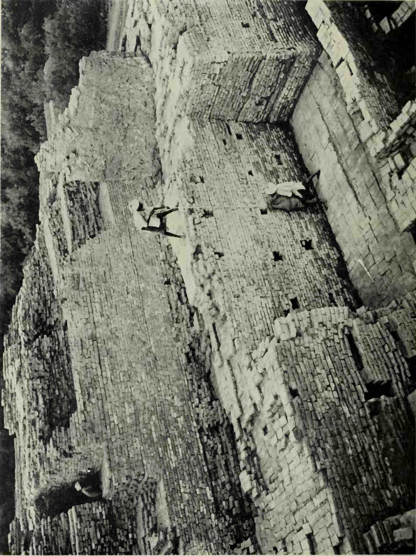
Mohenjo-daro: podium of the Great Granary from the north, showing alcove and platform for unloading vehicles. The uppermost figure is squatting in the end of one of the ventilation-passages which underlay the timber superstructure. The brickwork of the platform shows holes and grooves for timber bonding (excavated 1950) (p. 43).
