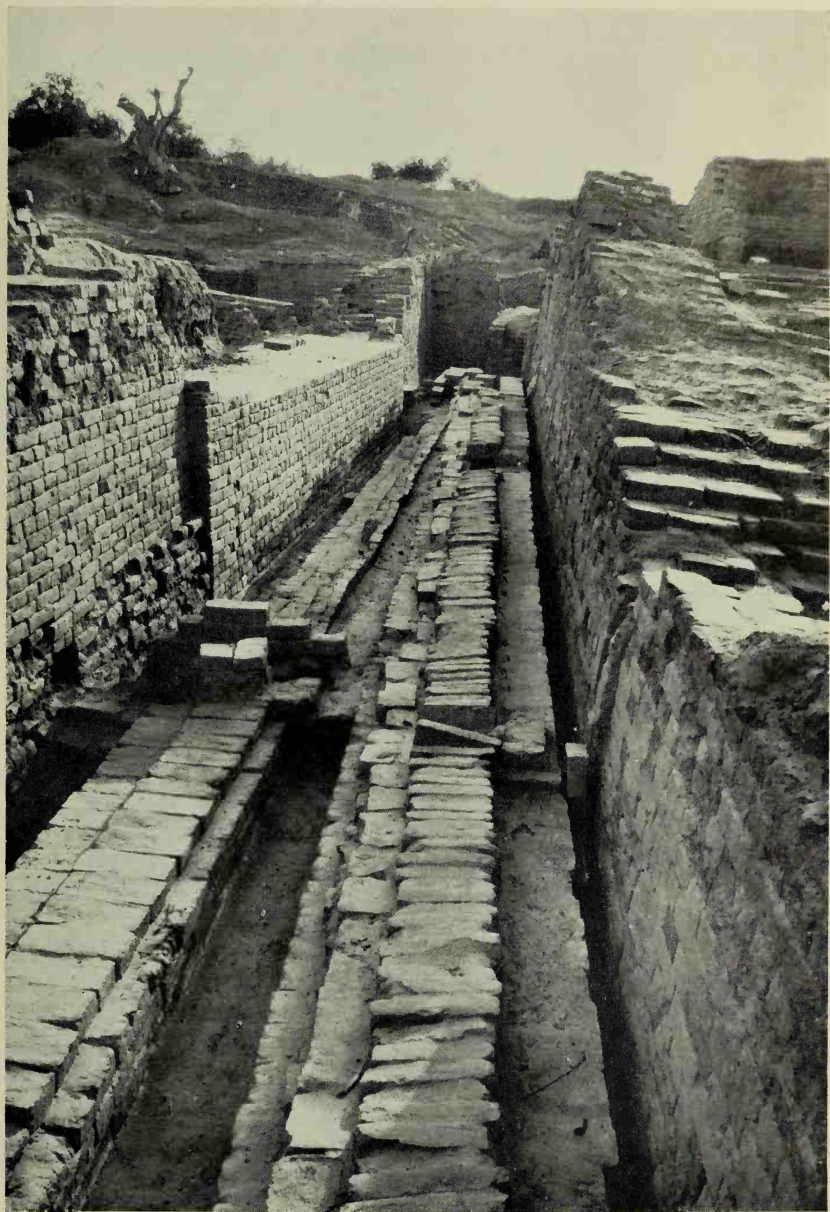
Mohenjo-daro: street with drains (p. 54).
