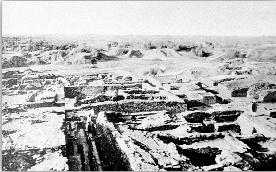
a. Building with small bathrooms, north of Great Bath, showing passage and drain, from W.
