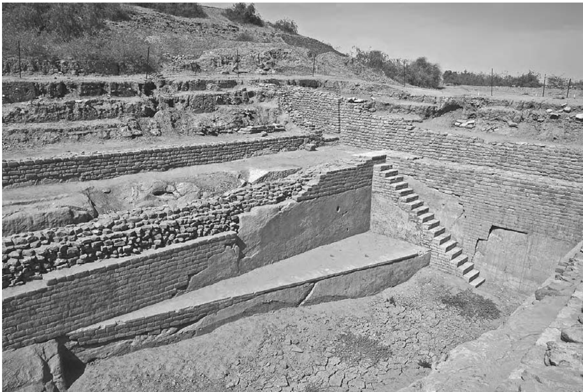
The enormous reservoirs are the most striking feature in the city of Dholavira. Steps down the side gave access to the water held in them. (Namit Arora)
