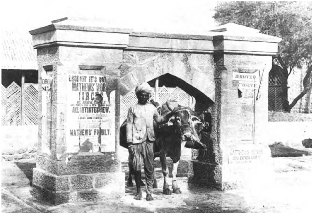
THE WATER WORKS - STAND FOR BULLOCK SERVICE
