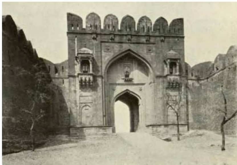
(b) ROHTAS FORT: THE SORAL GATE. (About A.D. 1340)
