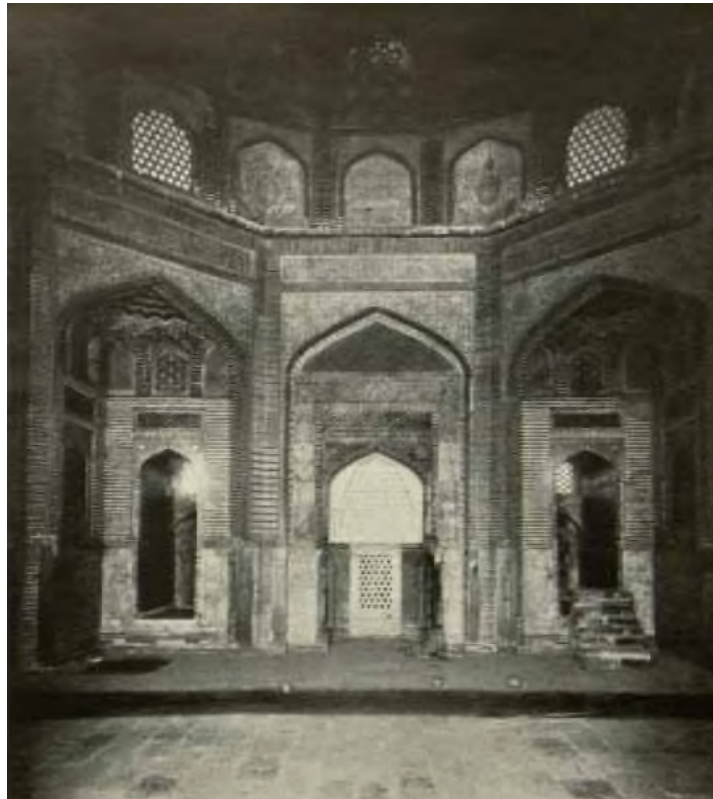
(a) THATTA: INTERIOR OF THE JAMI MASJID.
