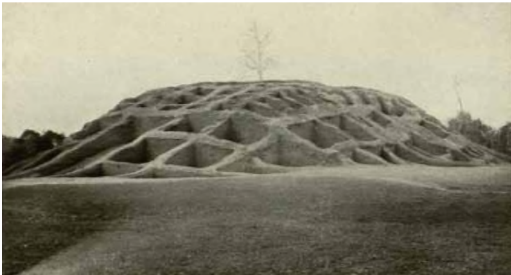
(b) MAHASTHAN: CELLULAR SUBSTRUCTURE OF A TEMPLE AT THE VILLAGE OF GOKUL (Possibly 7th century A.D.)
