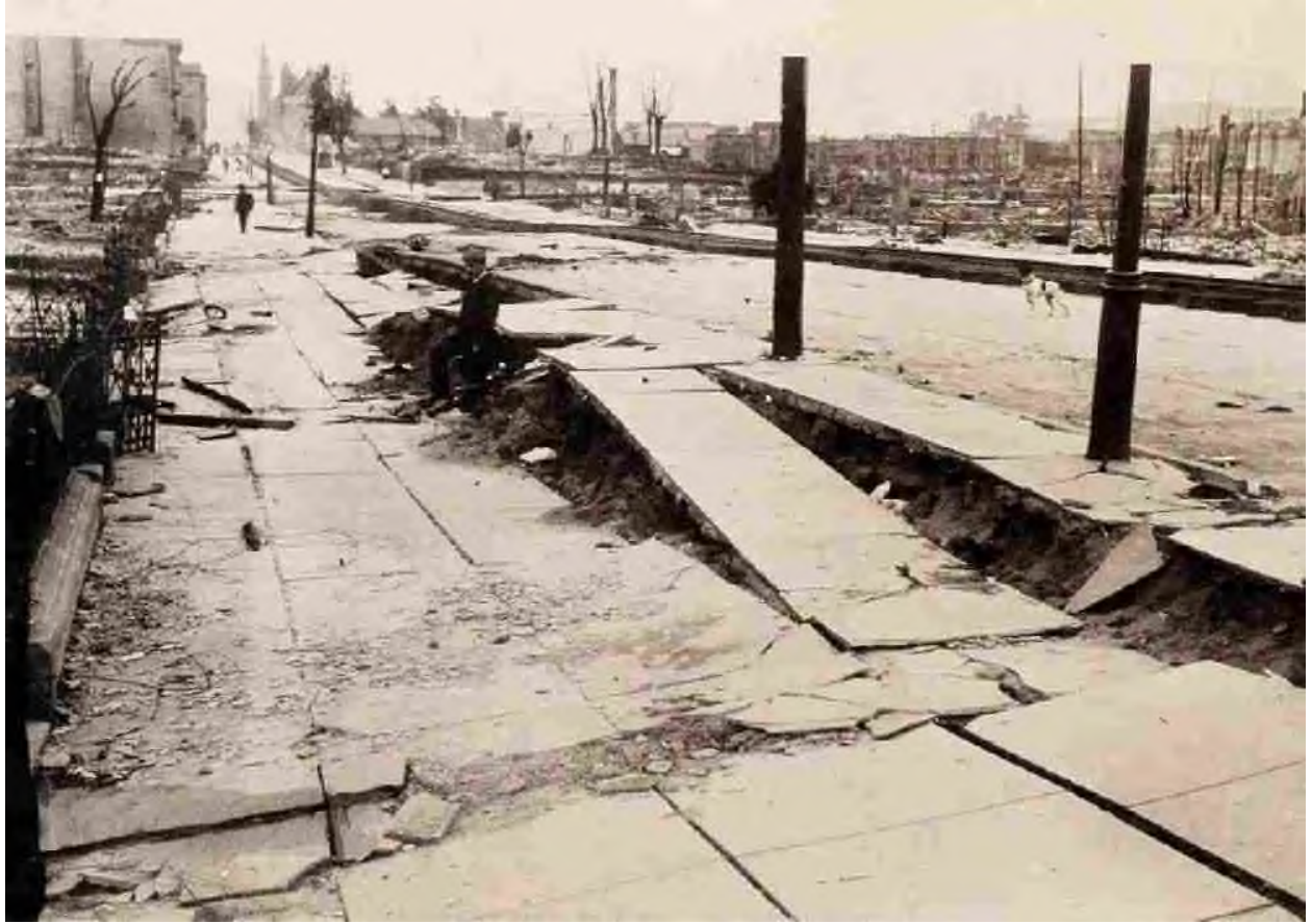
Break and Sink in Capp Street, Between Seventeenth and Eighteenth Streets, in the Mission District.
