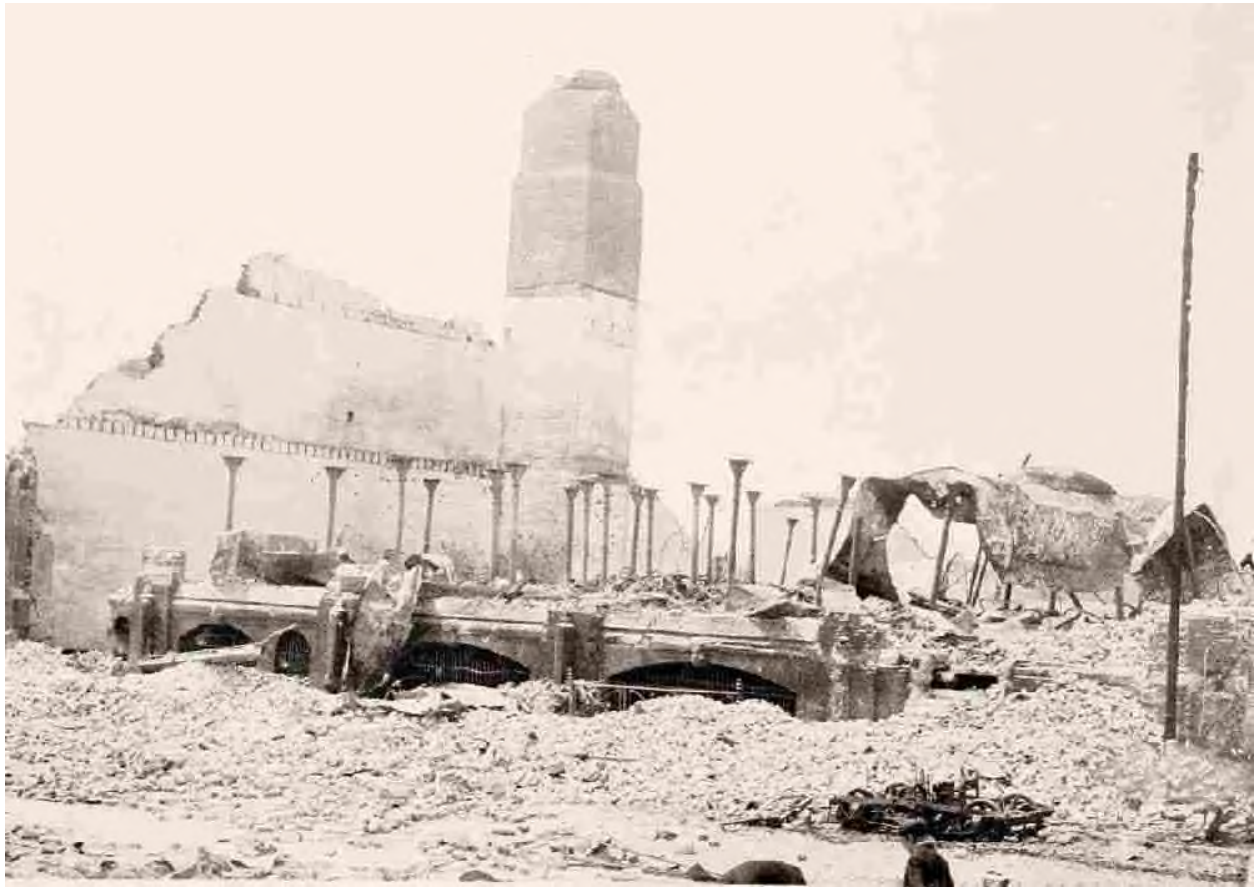
Cable Power-House ruins, corner California and Hyde Streets.
