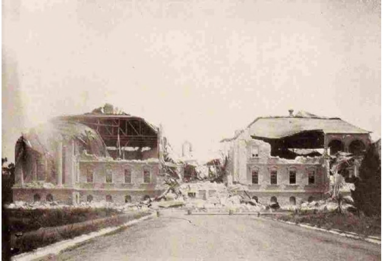
Effects of Shock: Wreck of New Gymnasium Building at Leland Stanford Jr. University, Palo Alto.
