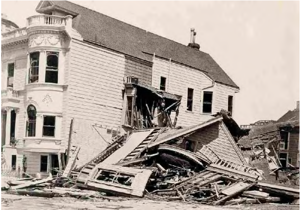
Effects of Shock on Frame Residence on Folsom, Near Seventeenth Street, in the Mission.
