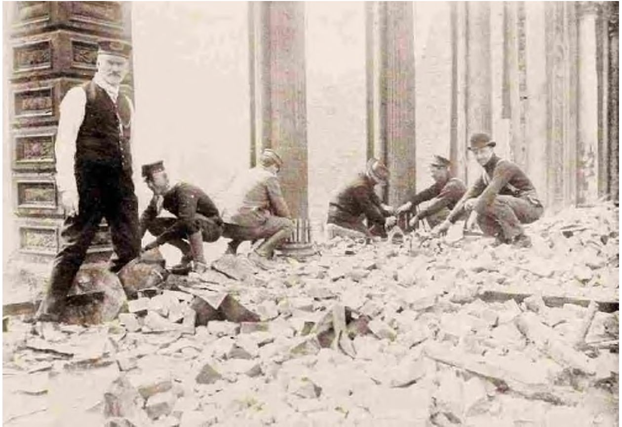
Dynamiting Crew of Regulars Destroying Buildings to Retard the Progress of the Flames.
