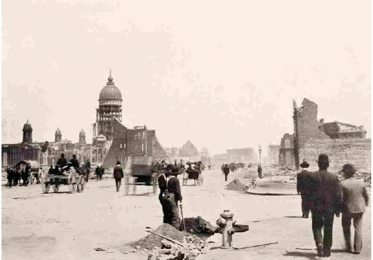
On Market Street at Ninth, One Week After the Fire; Refugees En Route to the Ferry; Men of the Board of Public Works Repairing the Water Mains.
