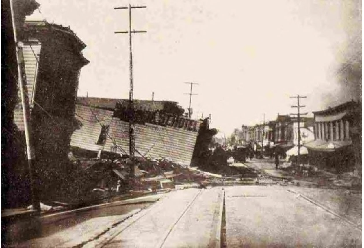
Effects of Shock: Wreck of the Valencia Hotel, Twentieth Street, in the Mission; Four-story Frame Structure, Sunk Two Stories Below Street Surface; Sixty-four Lives Lost.
