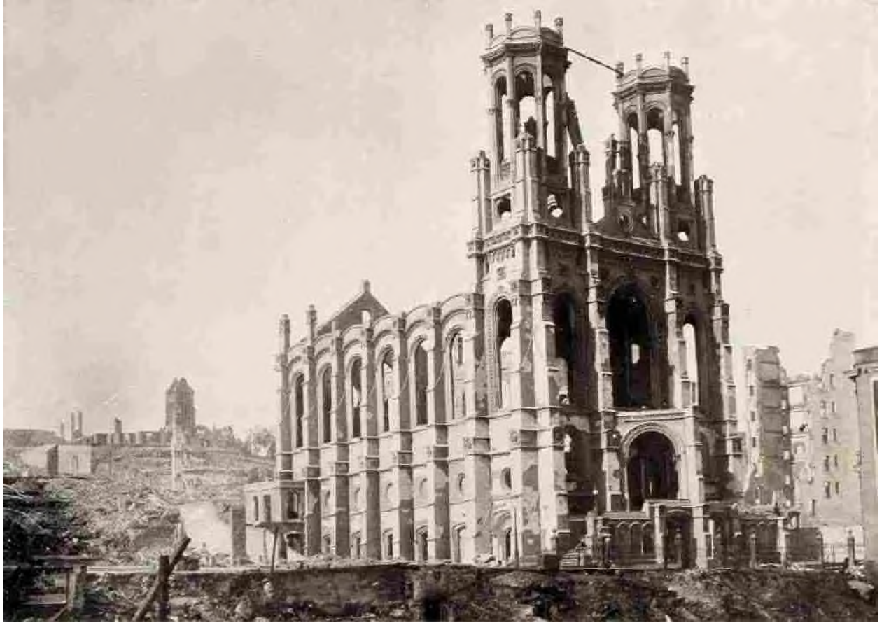
Ruins of the Large and Beautiful Temple Emanuel, on Sutter Street, Near Powell Street, Effects of the Earthquake and Flames.
