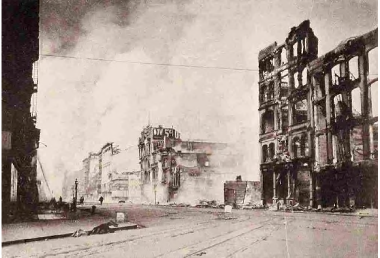
View from McAllister Street Looking East Along South Side of Market Street.
