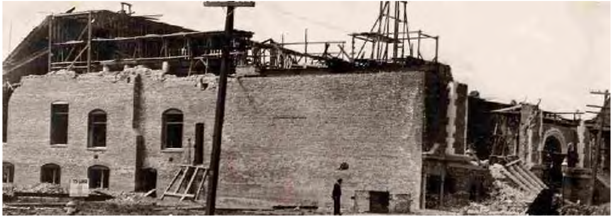
Effects of Shock on New Golden Gate Commandery, K. T., Building, in Course of Construction, Steiner and Sutter Streets.
