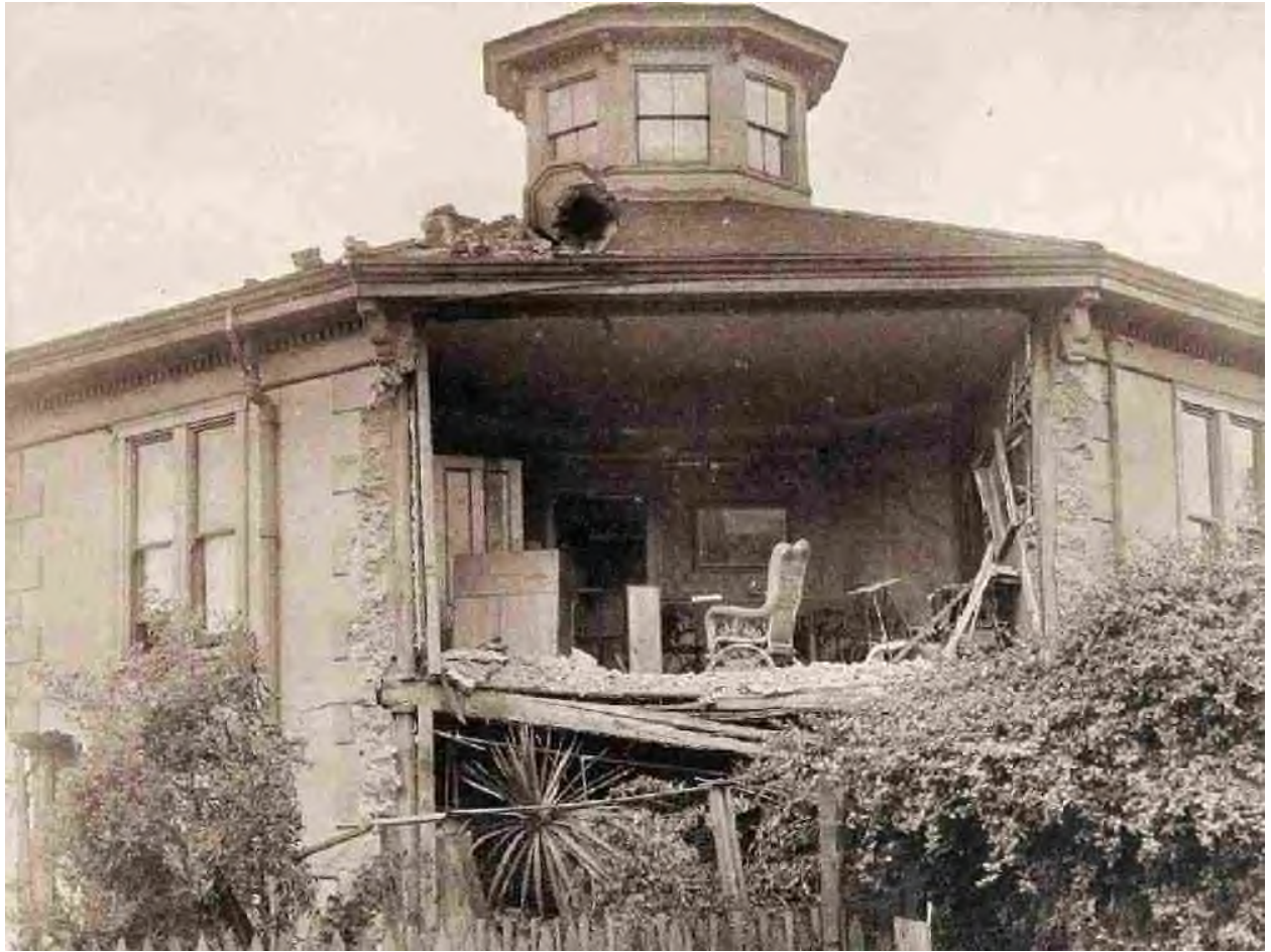
Effects of Shock on the "Octagonal House," a Residence on Gough Street, Near Union.
