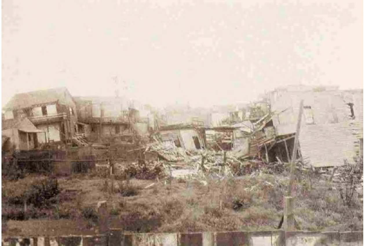
Effects of Shock: Wreck of Two-story Frame Homes on Brannan Street, Rincon Hill District.
