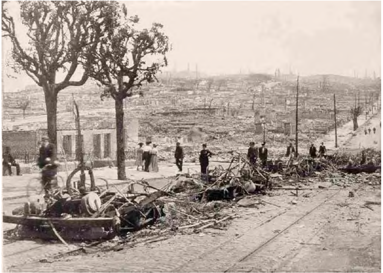
On California Street Near Van Ness Avenue; the Running-gears of the California Street Cable Cars, Which Were Burned Where They Stood.
