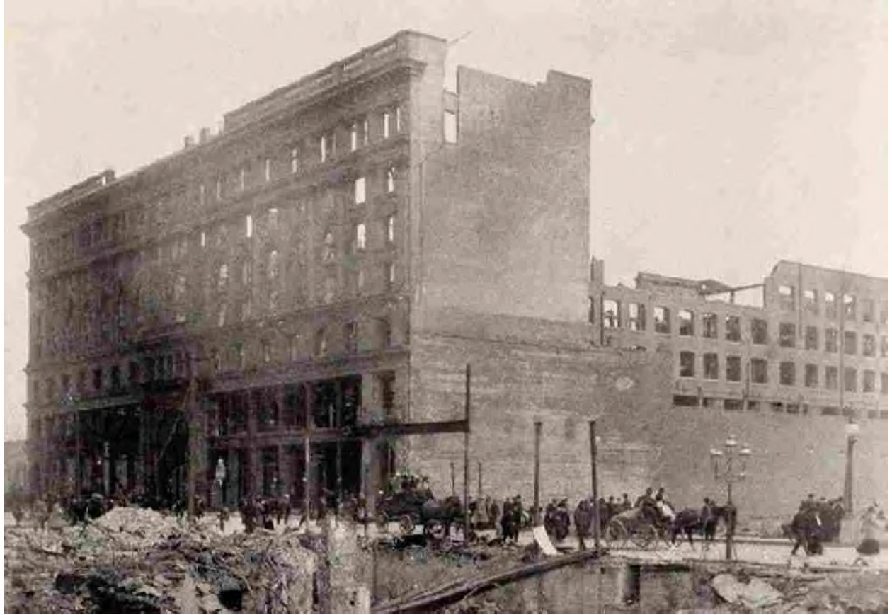
The Emporium Department Store, South Side of Market Street, One Week After the Fire; Showing the Rent in Wall at Top Story Caused by the Earthquake.
