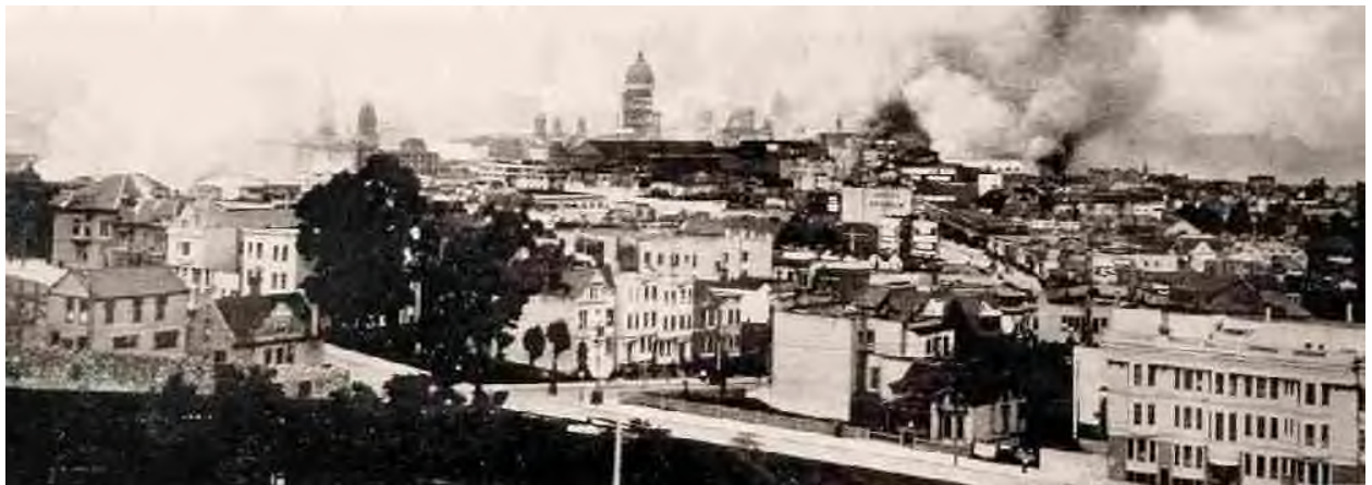
Fire Line at City Hall, Raging South of Market Street and on Golden Gate Avenue, First Day.
