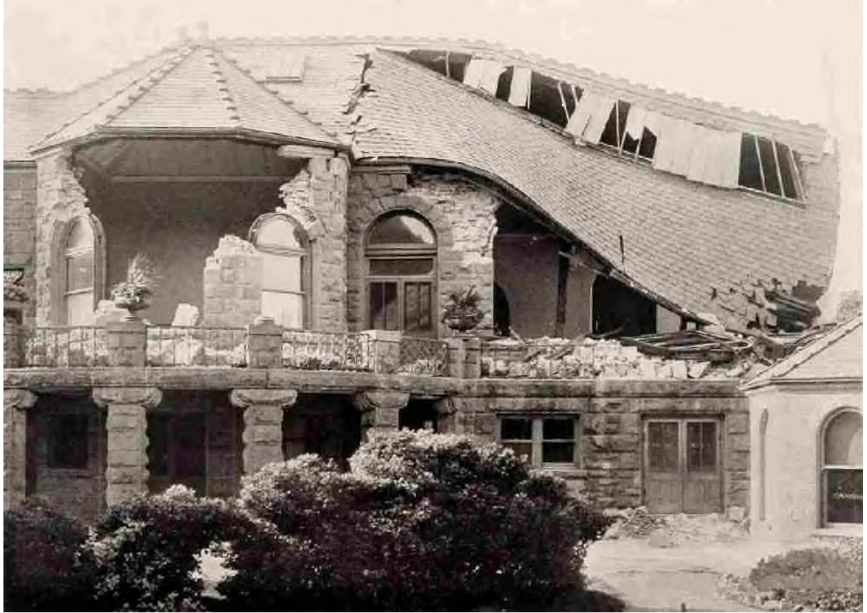
Effects of Shock: Total Wreck of the Children's Play-House, in Golden Gate Park; a City Building.
