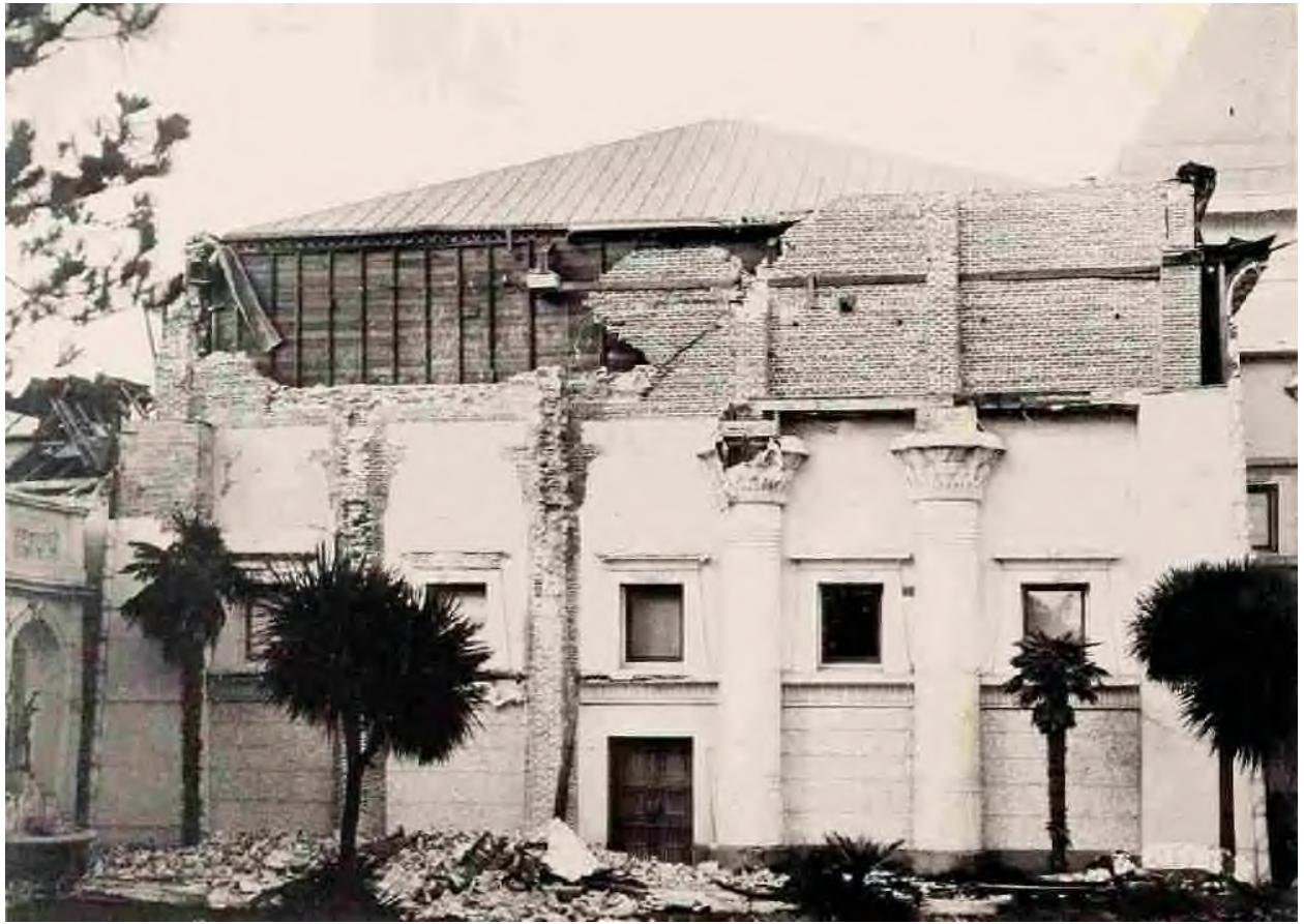
Effects of Shock on western side of Memorial Museum, Golden Gate Park, a Structure of the Mid-Winter Exposition.
