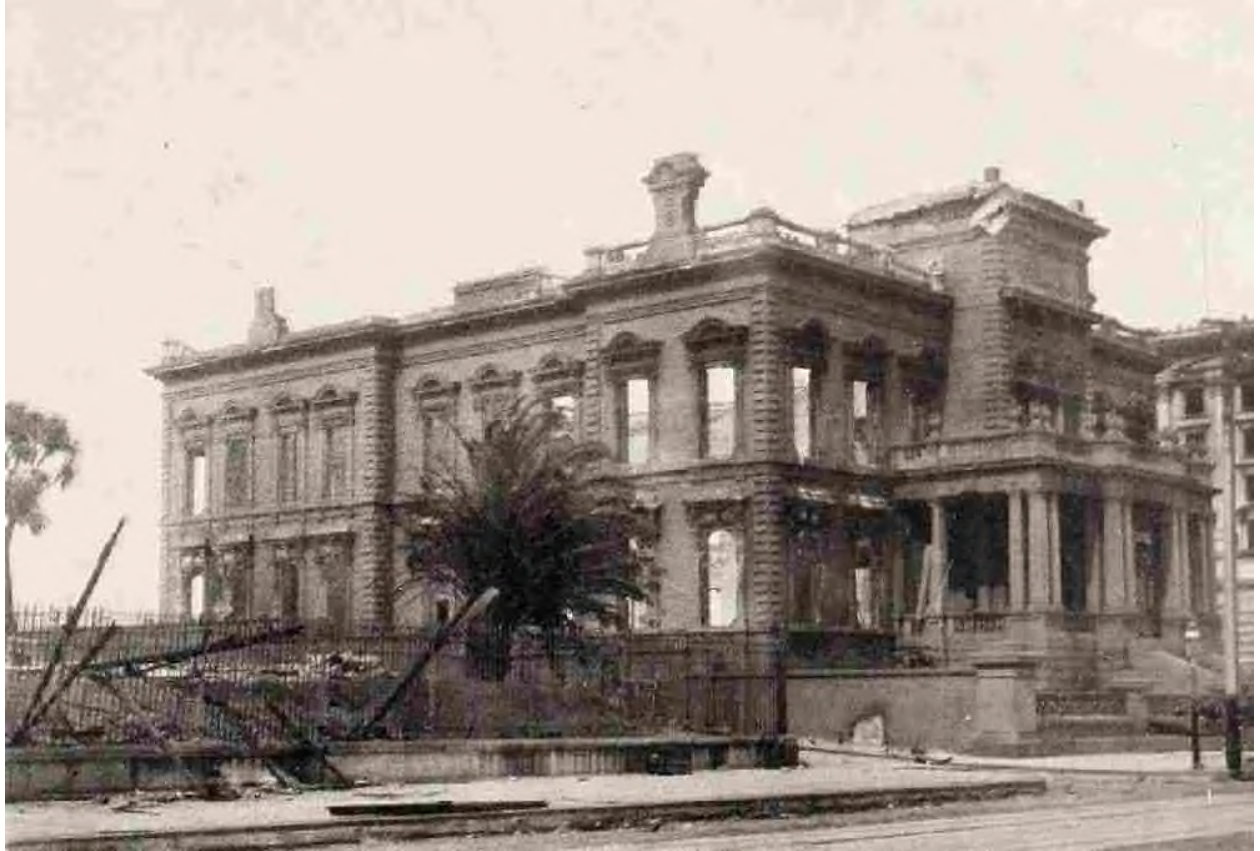
The Flood Mansion on Knob Hill, at California and Powell Streets; the Brown Sandstone in This Residence Was Brought Around the Horn in Sailing Vessels in the Early Fifties.
