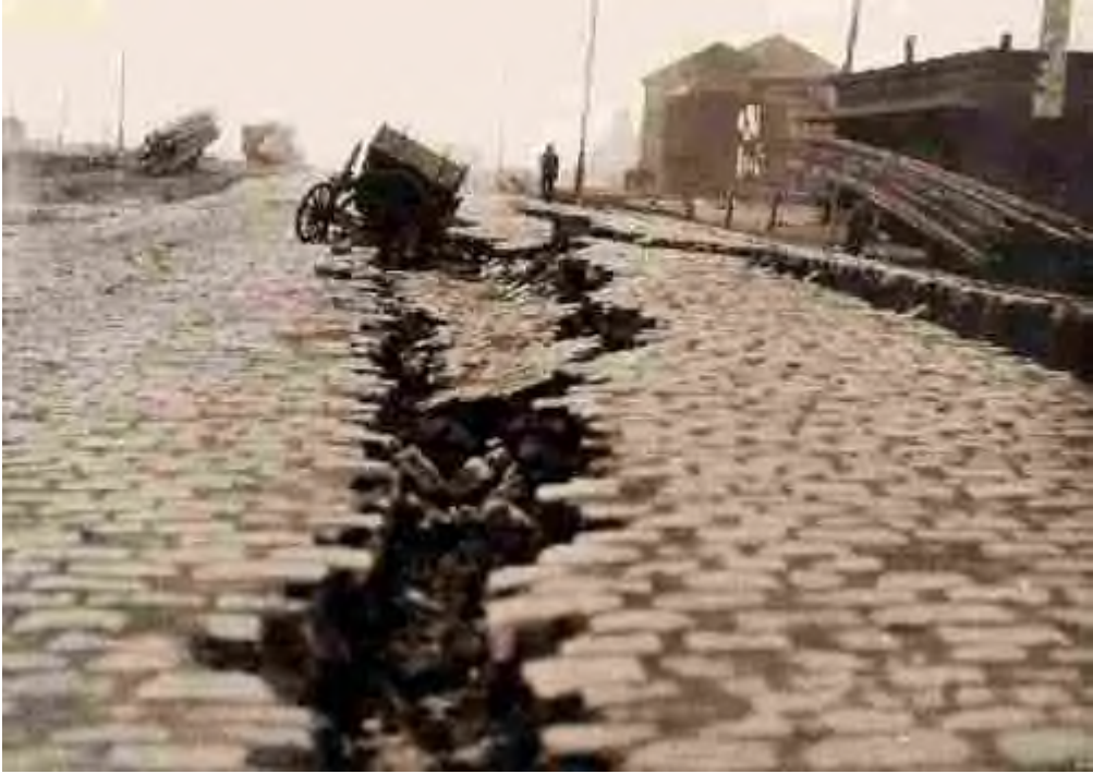
Break and Two-foot Sink in East Street, Near Ferry Building.
