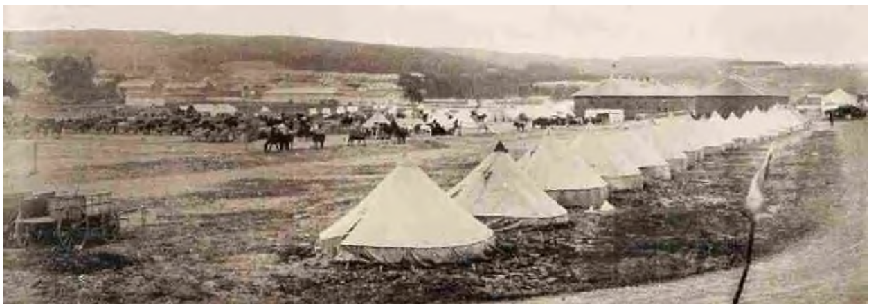
View showing the Cantonment on the Presidio Reservation, Cavalry and Artillery Barracks, and the Corral for the pack-trains used by the Army to transport the Relief Committee's supplies to the different camps.
