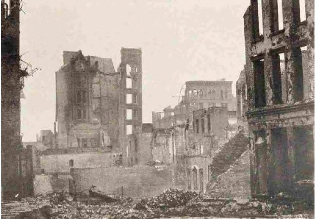
Looking East on Commercial Street, from Kearny to Montgomery, Showing the Pacific-Mutual Bank and Sub-Treasury.
