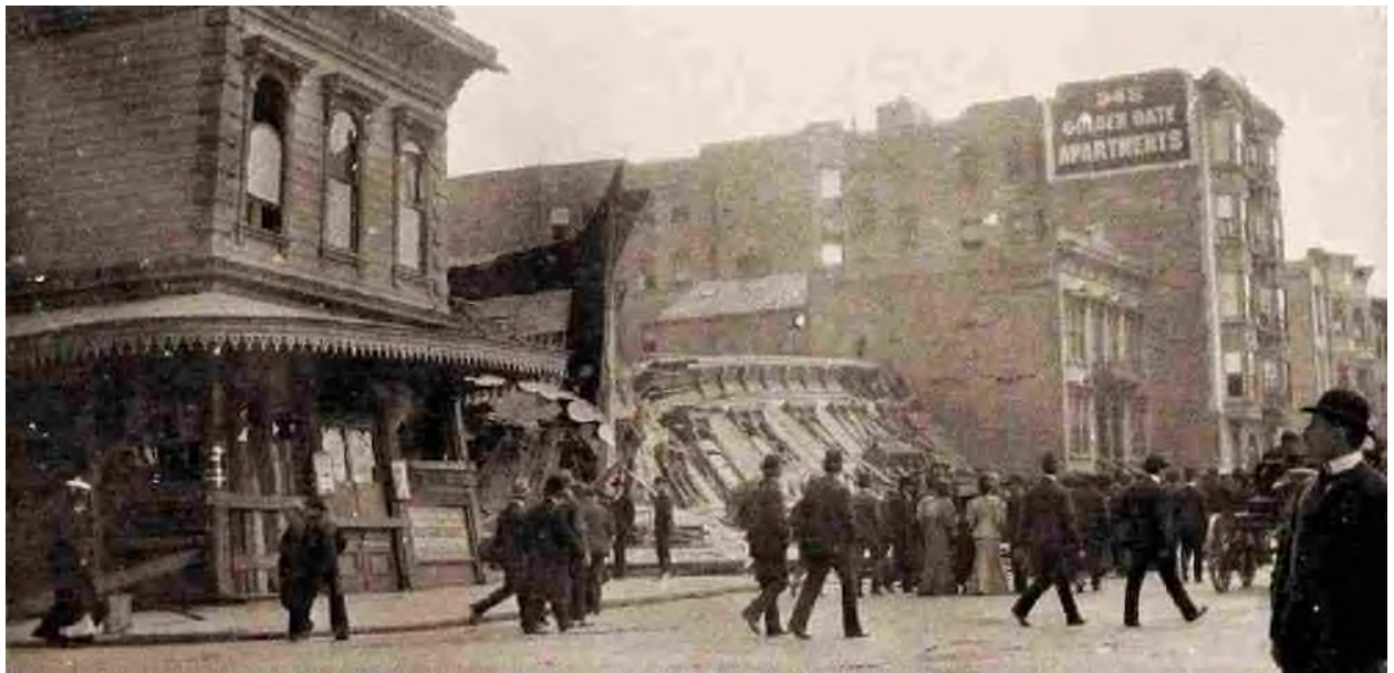
Effects of Shock on Two-story Frame Residence on Golden Gate Avenue.
