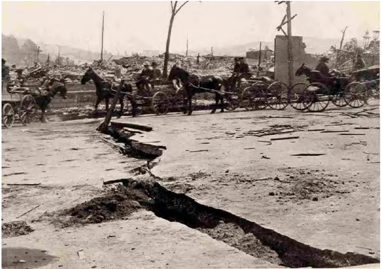
Break in the Asphalt Paving on Van Ness Avenue, Near Vallejo.
