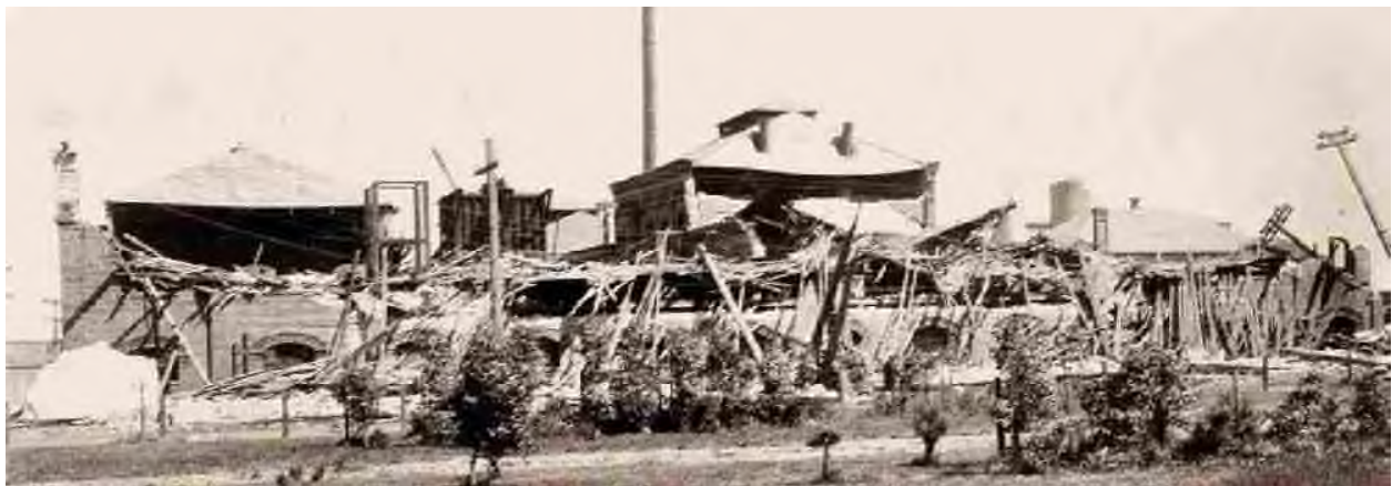
Effects of Shock on the San Francisco Gas and Electric Company's Power-House, Near Fort Mason.
