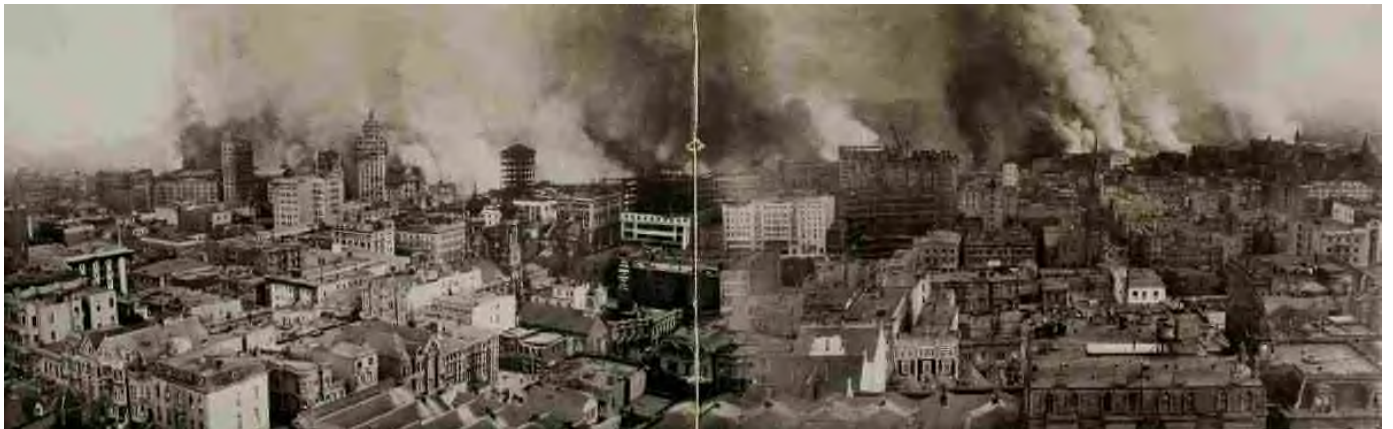
Fire Scene of the Entire District South of Market Street, from Stuart and Mission Streets to Sixth and Mission Streets; Also, Showing the Great Hotel, Newspaper and Retail Centers of the City North of Market Street at Noon of the First Day; on the Second Day All the District Shown in This View Was Entirely Flame Swept.
