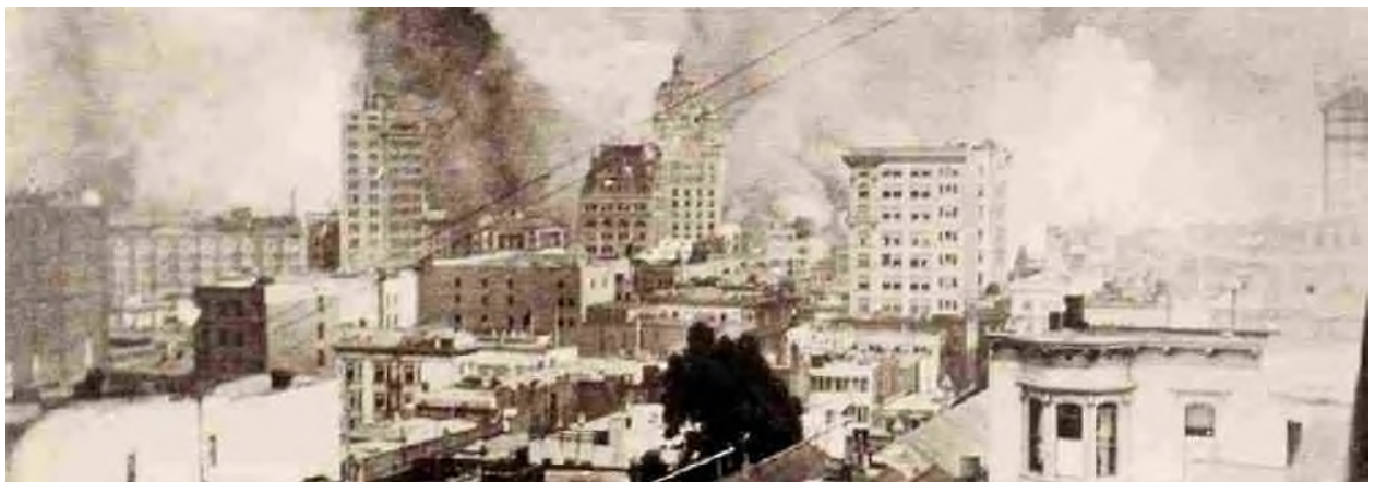
Fire Line South of Market, Early on First Day, Left to Right, Shows Palace Hotel, New Chronicle, Examiner and Call Newspaper Buildings, Mutual Savings Bank and New Shreve Office Buildings.
