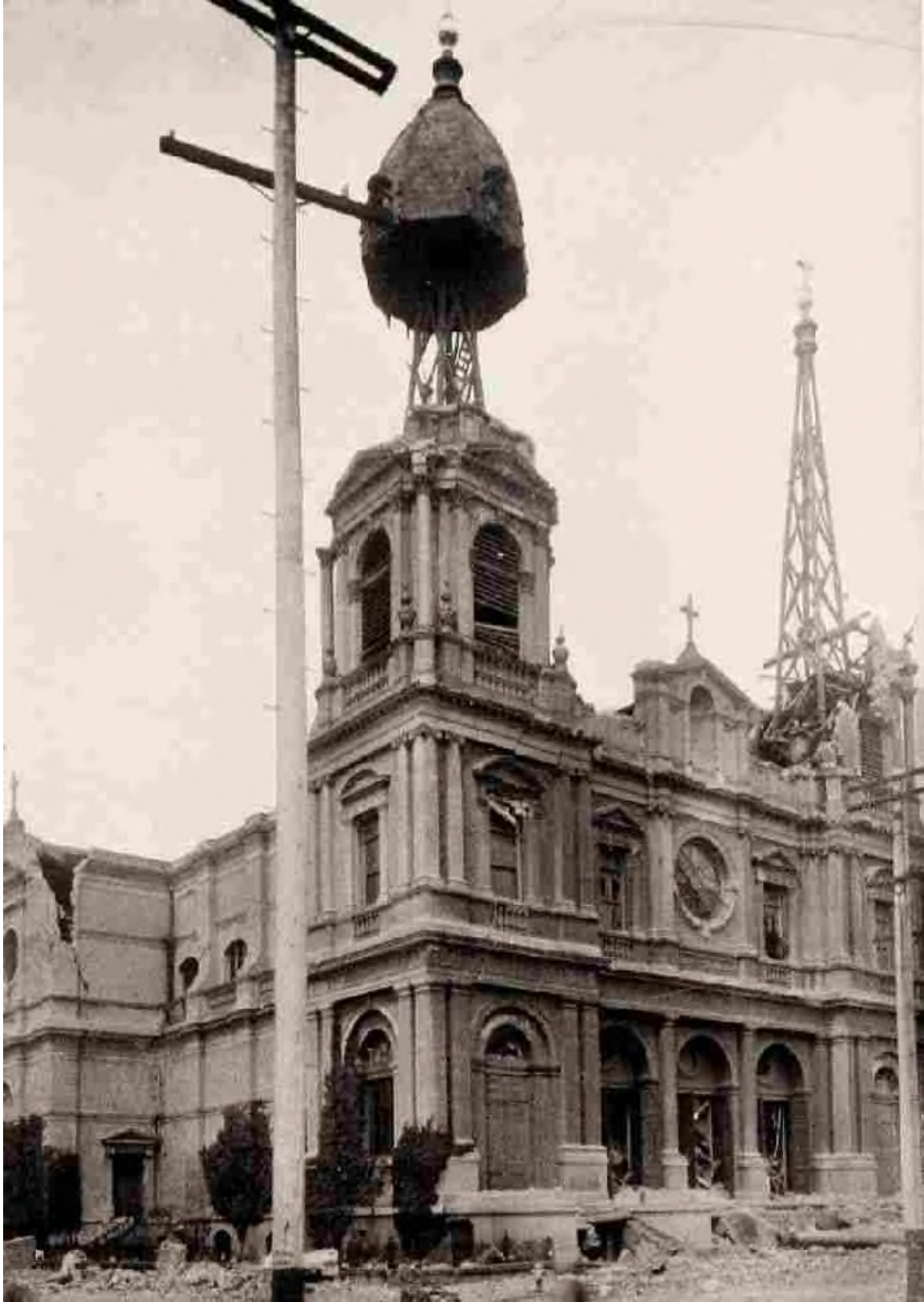
Effects of Shock on the Cathedral of St. Dominic, Steiner and Bush Streets.
