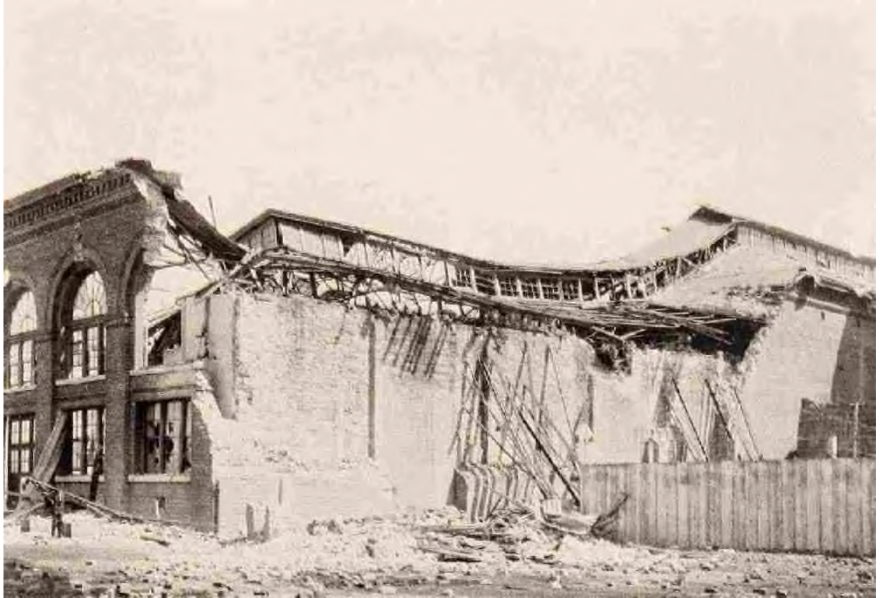
Effects of Shock: S. F. G. & E. Co.'s Gas-House, Near Fort Mason.
