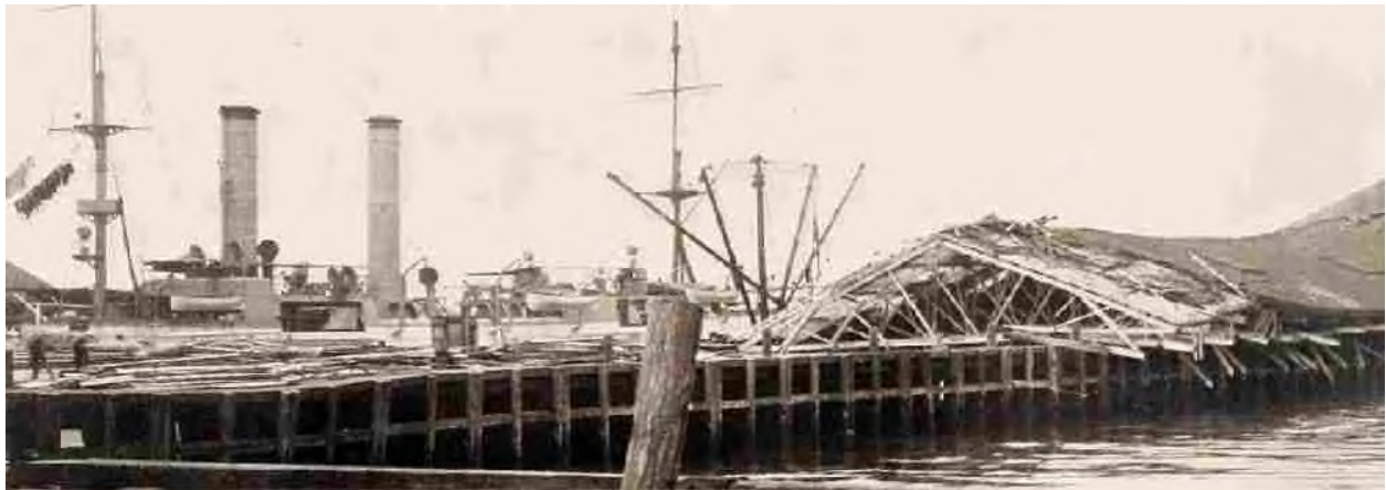
Effects of Shock: Wrecked Wharf No. 9; U. S. Cruiser Chicago Alongside; the Ship's Pumps Protected Much Wharfage Near This Point.
