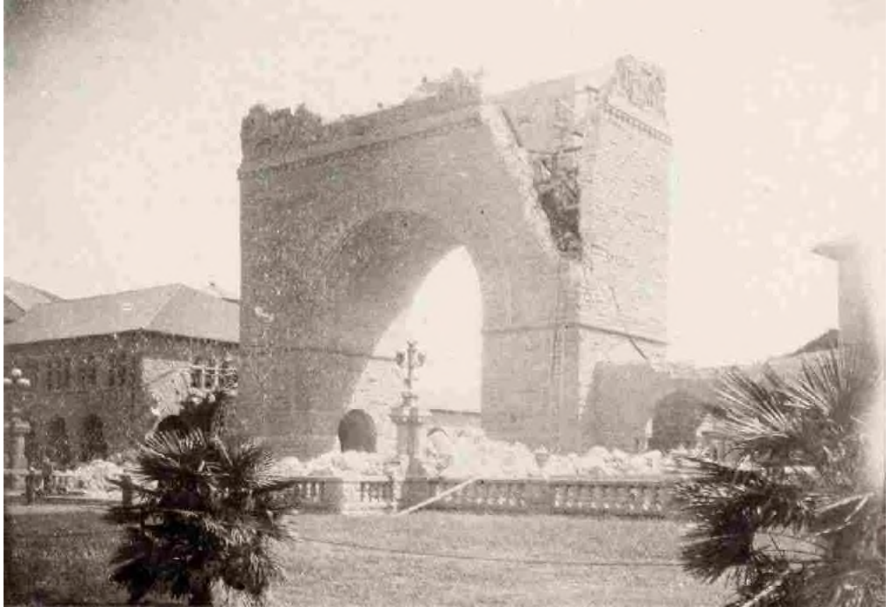
Effects of Shock: Wreck of Memorial Arch at Leland Stanford Jr. University, Palo Alto.
