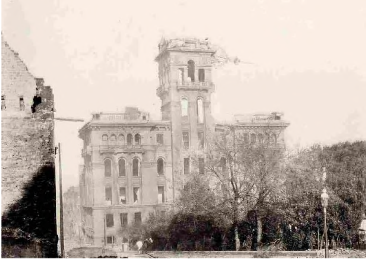
Hall of Justice, Kearny Street and Portsmouth Square showing shattered tower and gutted doors.
