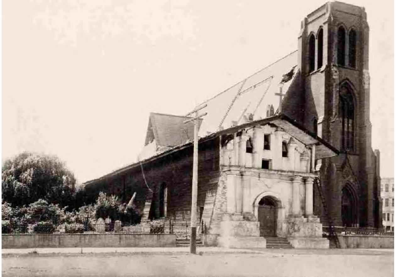
Effects of Shock on Dolores Mission, the Oldest Building in the City; Tower of the New Church, Which Will Have to Be Rebuilt.
