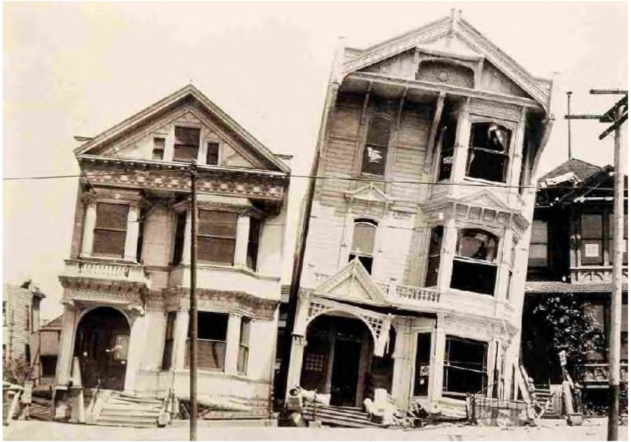
Effects of Shock on Two Frame Residences on Howard Street, Near Eighteenth, in the Mission.
