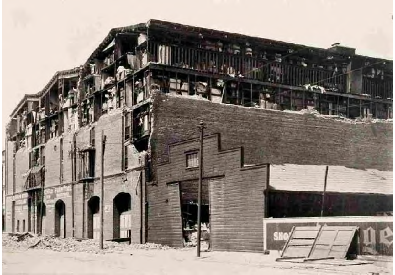
Effects of Shock on the Pierce-Rudolph Storage Warehouse, Fillmore Street.
