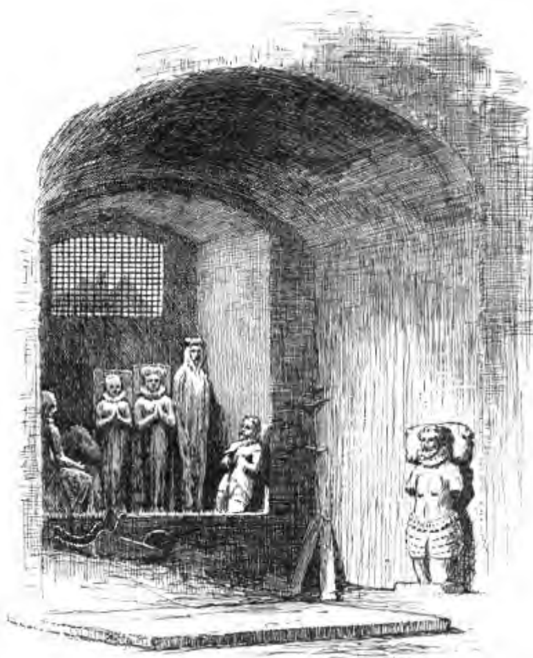
MONUMENTS OF ST. PAUL'S WHICH SURVIVED THE FIRE (EAST END OF THE NORTH CRYPT)
