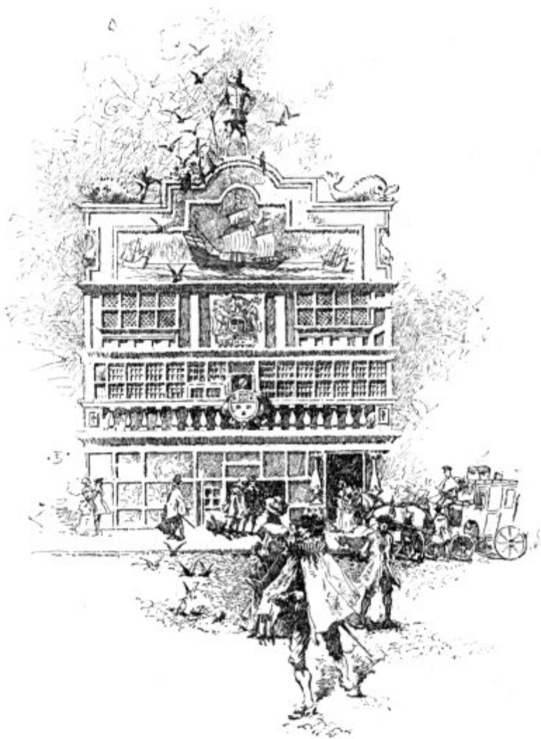
OLD EAST INDIA HOUSE
