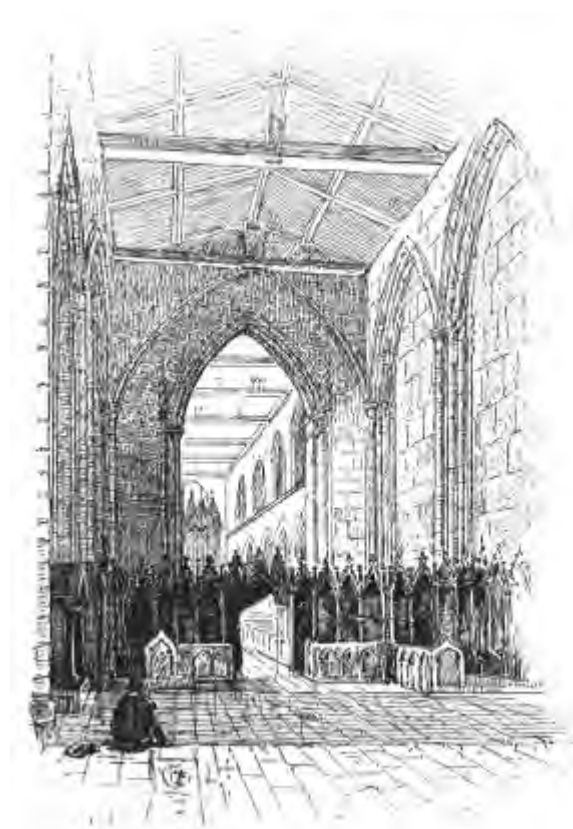
INTERIOR OF THE CHURCH OF ST. KATHERINE'S BY THE TOWER
