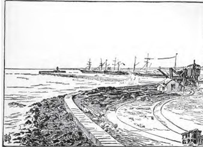
The Colombo breakwater, Ceylon
