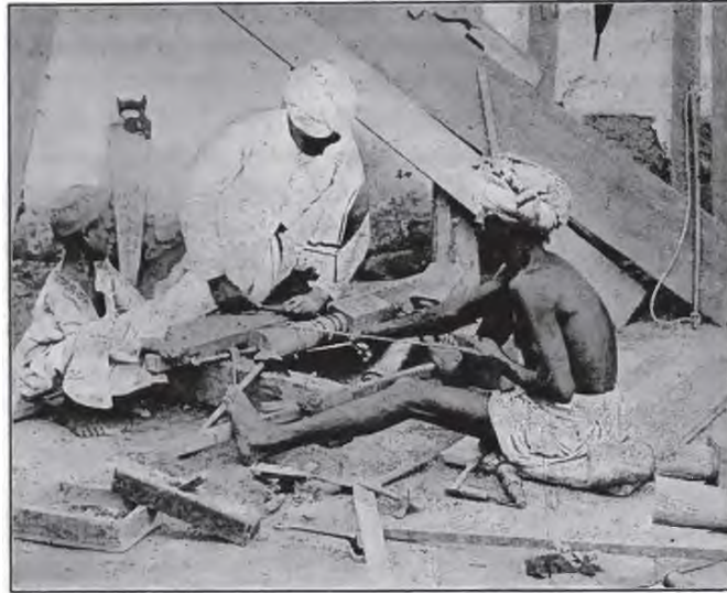
Indian carpenters at work.
