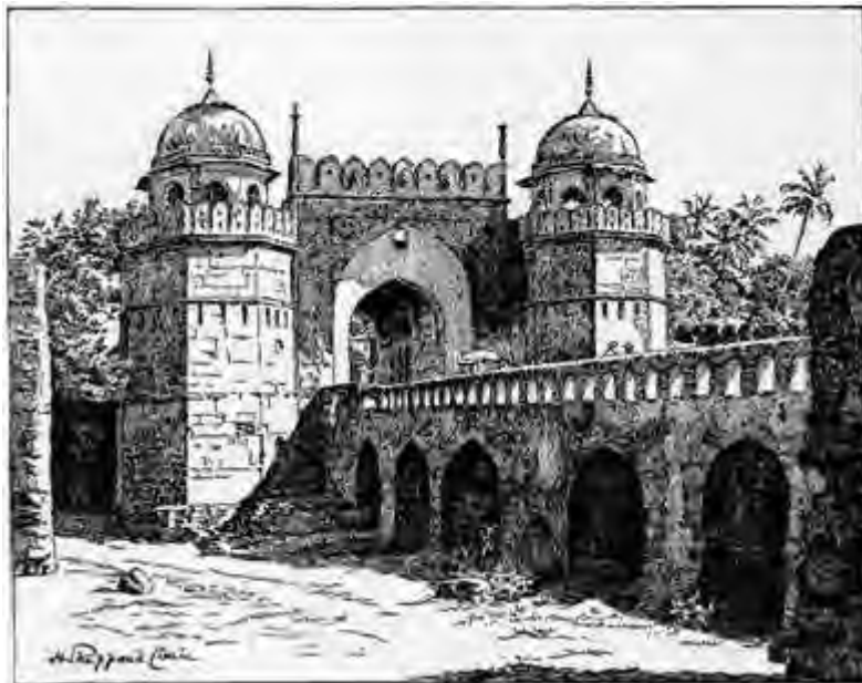
Mekka Gate at Aurungabad.
