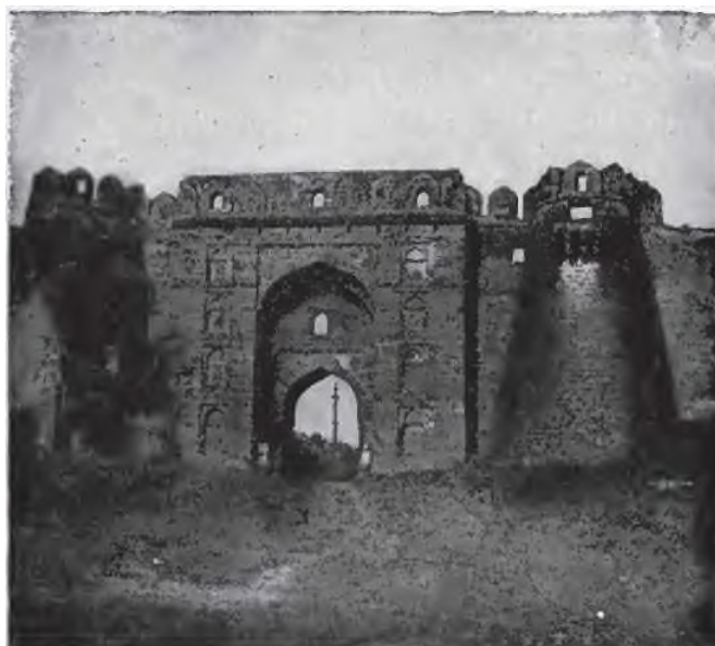
Fort of Jaunpur, east gate.
