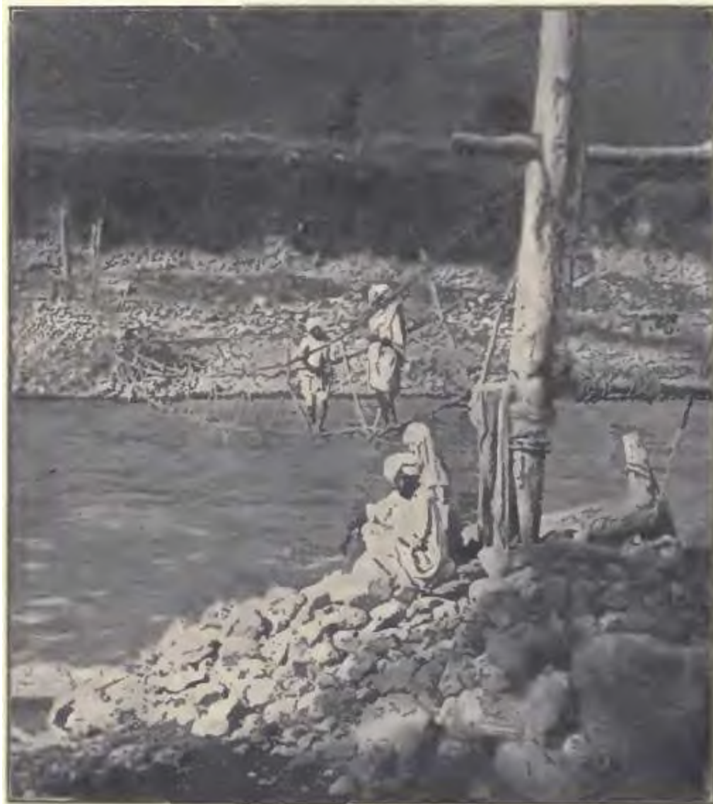
Rope bridge across the flooded Jihlam
