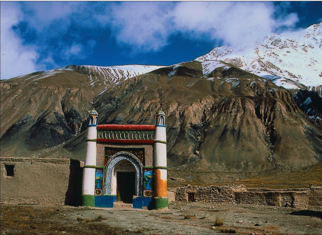
As Islam established itself along the Silk Road, mosques were built for travelers and local converts. This mosque in the Xinjiang province of China reflects the Central Asian influence in its design.
