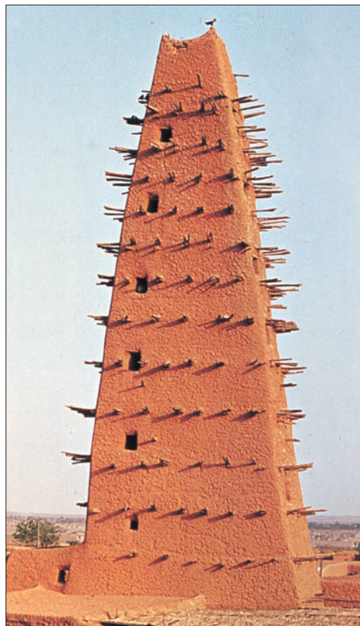
Originally built in the fourteenth century, the mosque at Agades, in Niger, is made of mud. Its structure is constantly renewed by workers bearing new mud who climb up the wooden posts that protrude from the sides and serve as scaffolding.
