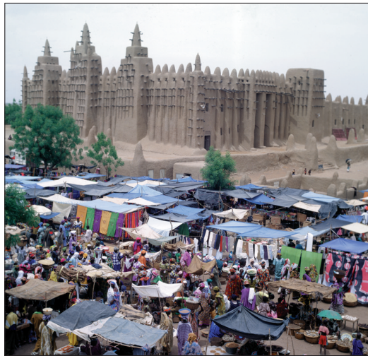
Mudbaked mosque at Djenne, Mali. Designed in the local vernacular style, the building fabric is constantly renewed from the material of which it is made.
