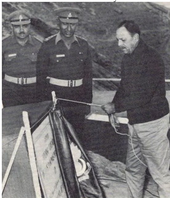
20a Opening the Srakha Gravity Dam, constructed by army engineers, near Quetta, 14 December 1962
