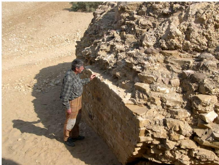
Fig. 11: Ranikot Fort. Sampling charcoals for radiocarbon dating from the collapsed pillar of Sann Gate (photograph P. Biagi)
