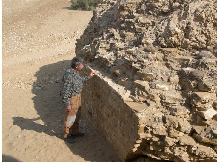
Fig. 3 - Ranikot Fort: the surface from which the charcoal sample was collected ( photograph by P. Biagi )
