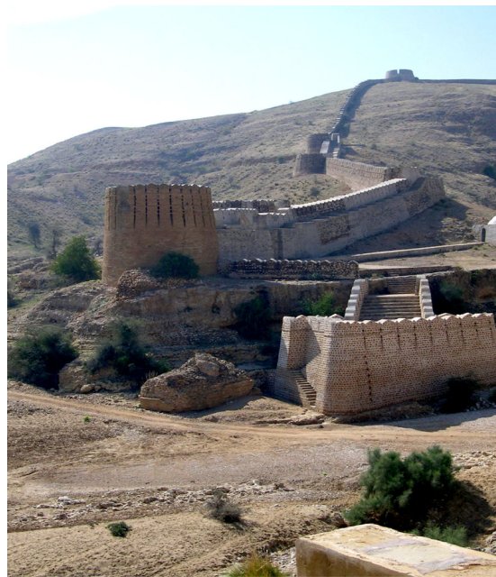
Fig. 2 - Ranikot Fort: the collapsed pillar at Sann (Eastern) Gate ( photograph by P. Biagi ).
